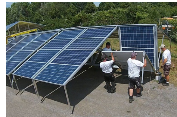
'the solar container': "ready in two hours to start producing electricity"
